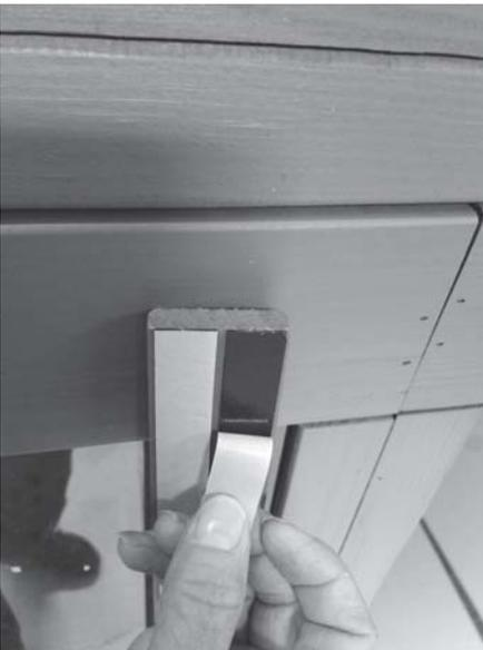
Align the trim to the top of the wall panel sections.
