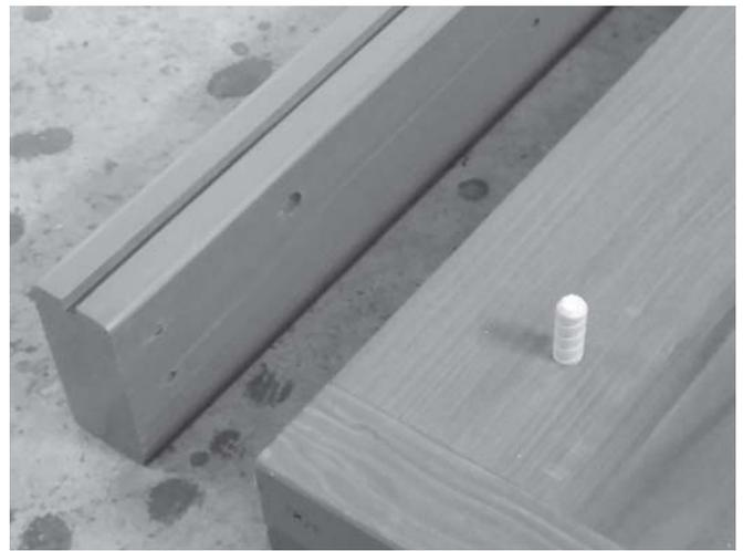
Insert dowels at the bottom end of the wall panel as shown above. These align the bottom frame.
