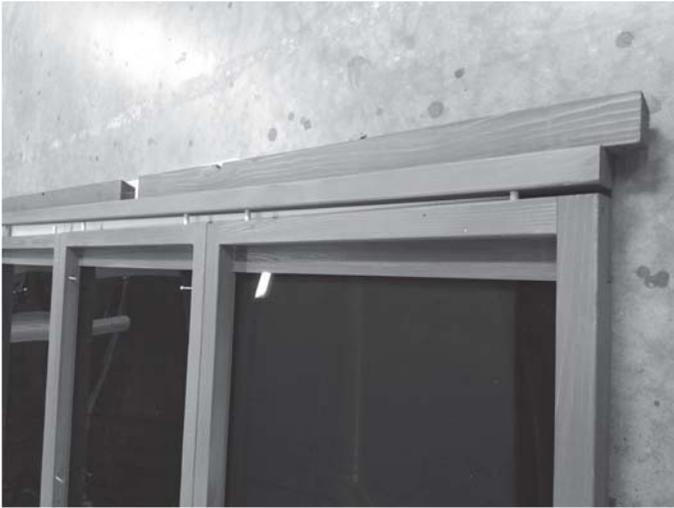
Insert the dowel pins in both the top and bottom as in previous instruction. Place the top and bottom frames onto the wall panels as shown and fasten using 2 1/2 inch wood screws.
