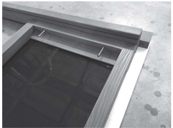
Fasten the wall panels to the top frame using 2 1/2 inch wood screws as shown above. Smaller panels use two screws per panel. Larger panels use three screws per panel..
