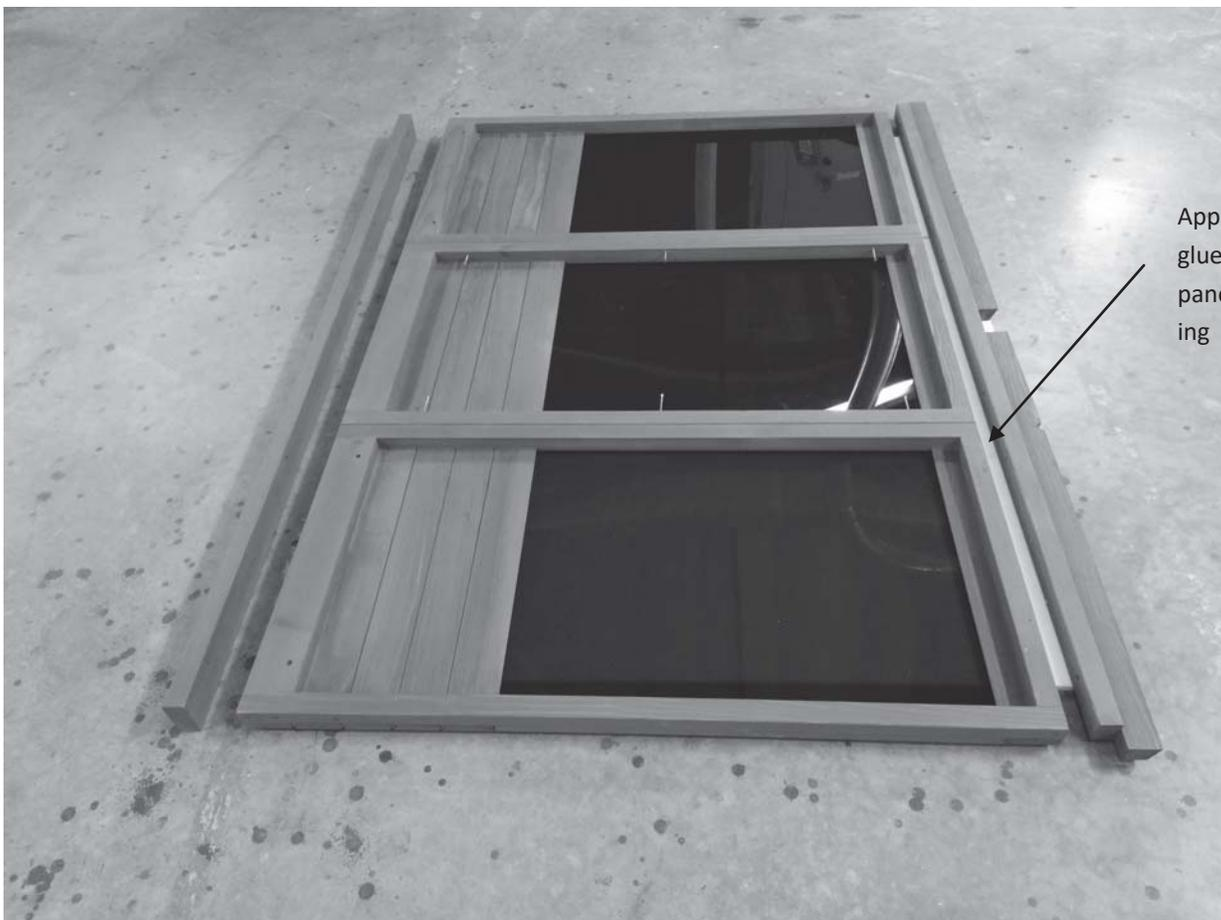
Apply a bead of glue to top of wall panel before joining
